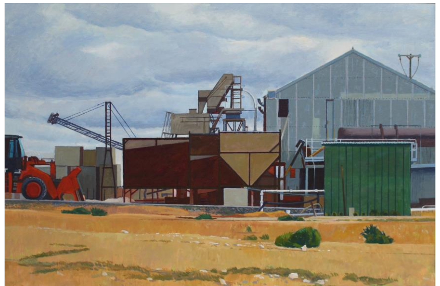
Buildings salt works near Langhorne Creek 2020
